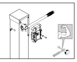
**07.** Taking care not to lose control of the boom pole, clamp it onto the pole mount base with the pole mount outer cover.
